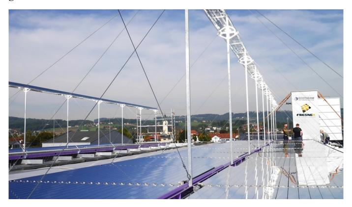
Together with the company ECOTHERM AUSTRIA, FRESNEX enabled the integration of a 200 m<sup>2</sup> solar field into an existing steam system.
